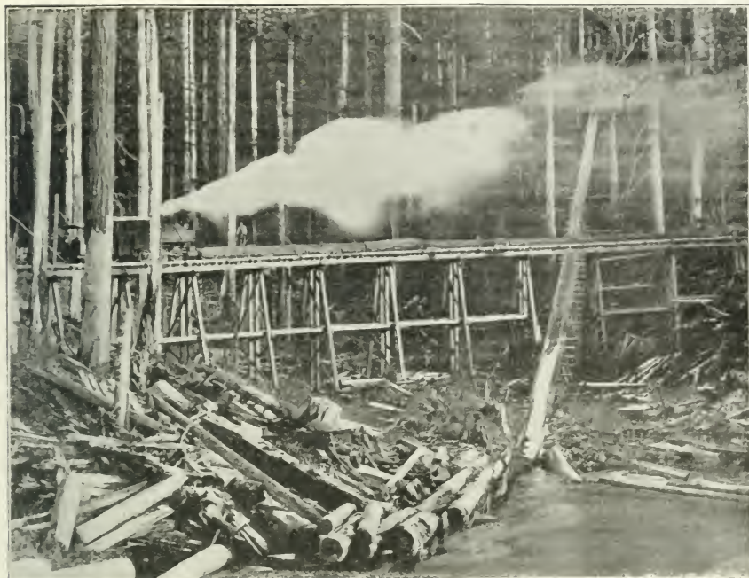
6.—"THE LOGS ARE PULLED ALONG OVER THE SLIDERS, NO ROLLING-STOCK BEING EMPLOYED."
