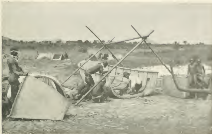
A STEEL BOAT, BROUGHT UP IN SECTIONS FROM ENGLAND, BEING BOLTED TOGETHER. From a Photo. by Mr. de Winton.
