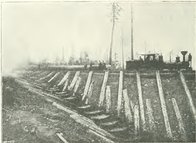
A LOCOMOTIVE HAULING A TRAIN OF LOGS--IN THE FOREGROUND IS SEEN THE UPPER END OF A "CHUTE" DOWN WHICH THE LOGS SLIDE INTO THE RIVER. [Photo.]
