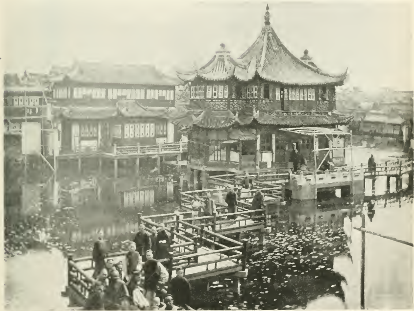
EVIL SPIRITS ON THE BRIDGE, LAZIED THEM AS BEING EASY, THEREFORE THIS QUAINZ BRIDGE (AT SHANGHAI) WAS BUILT IN ZIG-ZAG FASHION. (Photo.)
