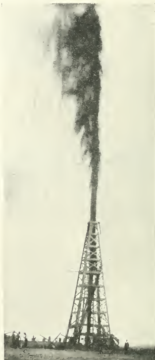
5.—THE LARGEST OIL-WELL IN THE WORLD—IT SPOUTS AT THE RATE OF 25,000 BARRELS A DAY, AND RISES NEARLY 200FT. From a (Photo.) INTO THE AIR. (Photo.)
