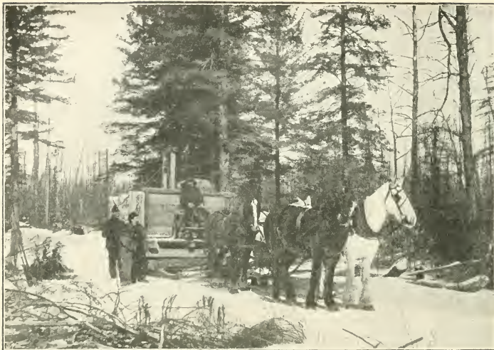
8.—LAYING AN ICE RAILROAD.—THIS PHOTOGRAPH SHOWS THE TANK FROM WHICH THE "RAILS" OF THE ICE-ROAD ARE "LAID."
