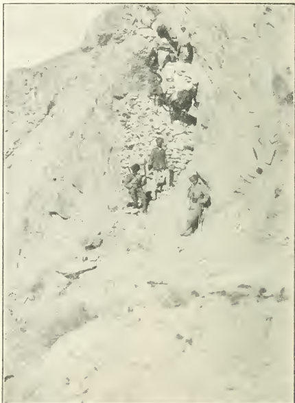
A BAD PART OF THE "ROAD" NEAR CULMIT, FROM A] IN HUNZA. [Photo
