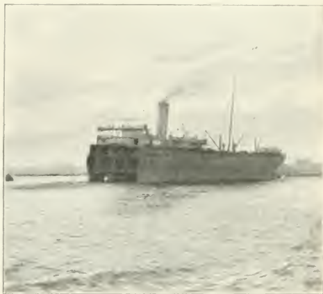
11.—THIS SHIP WAS WRECKED, BUT THE ENTERPRISING SALVAGERS CUT OFF THE REAR HALF, TO BE BUILT UP FIRST, AND LEFT A NEW FORWARD ON TO IT.
