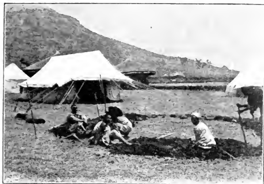
HOW ABYSSINIANS COMMENCE TO BUILD THE FOUNDATIONS OF A HOUSE. [Photo.]
