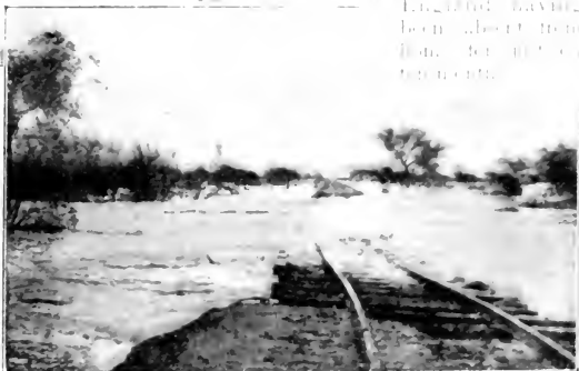
FIGURE 12. THE WASHING OF RAILS ON THE RAILWAY. [Photo.]
