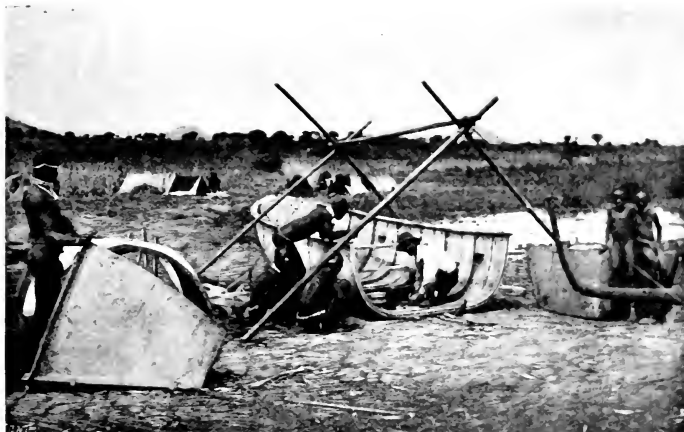
A STEEL BOAT, BROUGHT OUT IN SECTIONS FROM ENGLAND, BEING PUT TOGETHER. From a Photo. by Mr. R. Whitmore.
