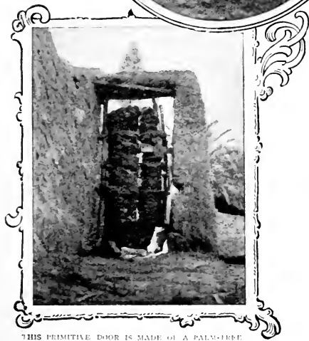
"THIS PRIMITIVE DOOR IS MADE OF A PALM-FERN TRUNK SPLIT INTO HALVES AND TIED TOGETHER." From a Photo.
