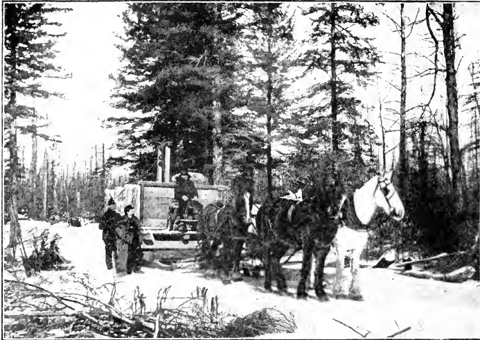
8.—LIVING AN ICE RAILROAD.—THIS PHOTOGRAPH SHOWS THE TANK FROM WHICH THE "RAILS" OF THE ICE-ROAD ARE "LAID."
