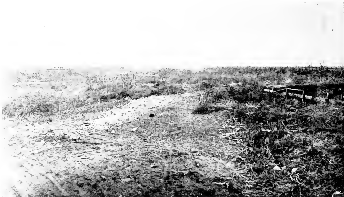
THE RIDGES IN THE CENTRE OF THE PHOTOGRAPH SHOW WHERE "MILITARY GOVERNOR" W. H. NILES CONSTRUCTED HIS RIFLE-PITS.
