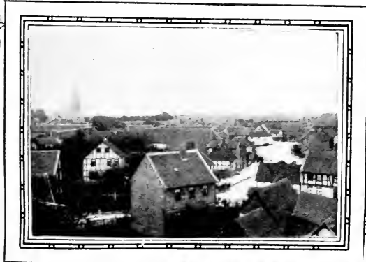
GENERAL VIEW OF STROBECK. From a Photo.
