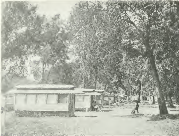
SUMMER DWELLINGS AT WAUKESHA BEACH, WISCONSIN—THEY WERE FORMERLY TRAM-CARS AND MAKE IDEAL ABODES. [Photo.]
