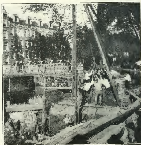
From a DRIVING IN PILES WITH THE "BEETLE." [Photo.]
