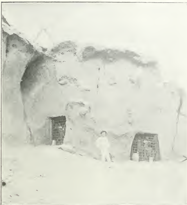
From a] THE GAOL AT SANTA ROSALIA, MEXICO—IT IS CUT OUT OF THE SOLID ROCK.
