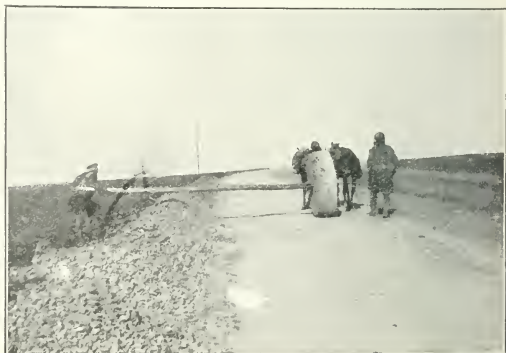
ROAD-MAKING IN THE EAST—"THE MAN STEERING THE ROLLER IS SECURELY STRAPPED TO HIS POLE, AND WERE THE STONE TO TOPPLE OVER HE WOULD BE HOISTED HEAVENWARDS." [Photo.]
