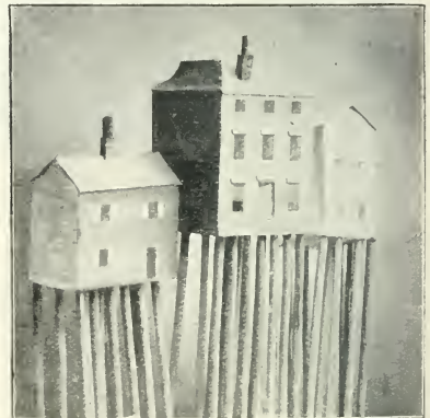
THE HOUSES IN THE GEISER-STRAAT, WHICH WERE LEFT PERCHED HIGH IN THE AIR—FROM A MODEL IN THE WATERSTAAT MUSEUM. [Photo.]
