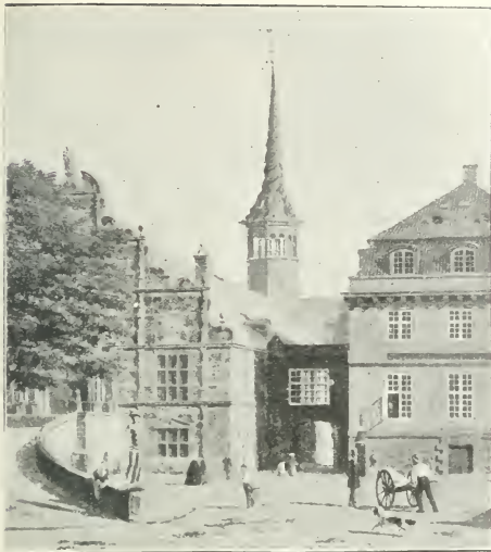
TO THE RIGHT IS THE OLD BANK, TO THE LEFT THE ROYAL EXCHANGE —IT WAS IN THE GALLERY BETWEEN THAT THE TWO CLERKS FIRST MET THE BLOODHOUNDS.
