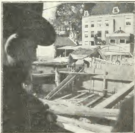
PUMPING OUT THE WATER PRIOR TO PILE-DRIVING. From a Photo.
