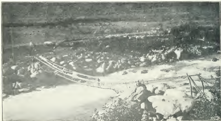
AN INDIAN "JOULA," OR NATIVE SUSPENSION BRIDGE—IF TWO PEOPLE GOING IN OPPOSITE DIRECTIONS MEET IN THE MIDDLE ONE OF THEM HAS TO RETRACE HIS STEPS. [Photo.
