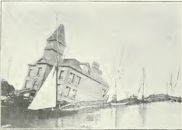
OCCASIONALLY THE "STILTS" SUPPORTING A HOUSE GIVE WAY, AND THEN THE BUILDING SUBSIDES INTO THE MUD—THIS PHOTOGRAPH SHOWS A PALATIAL RESIDENCE WHICH COLLAPSED SOME YEARS AGO.
