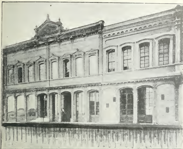
From a] A WAREHOUSE IN AMSTERDAM, SHOWING THE FOUNDATION OF PILES. [Photo.
