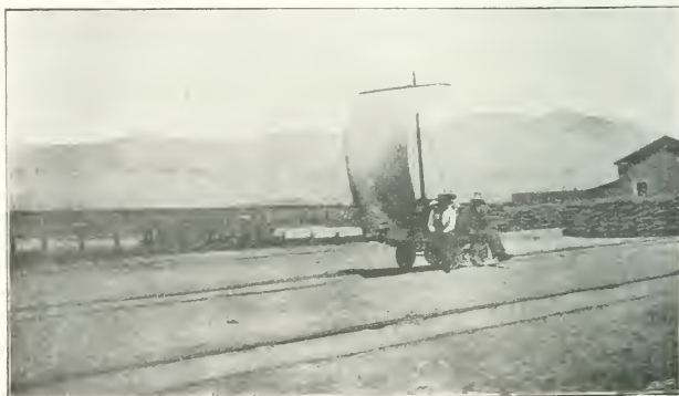
From a TROLLEY TRAVELLING ON THE FERRO CARRIL TALLAL, IN CHILE. [Photo.]
