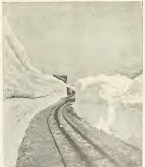
A SNAPSHOT ON THE 14,000-FT. RAILWAY UNDER THE ROCKS OF SWITZERLAND. (2 FT. 11 IN.)
