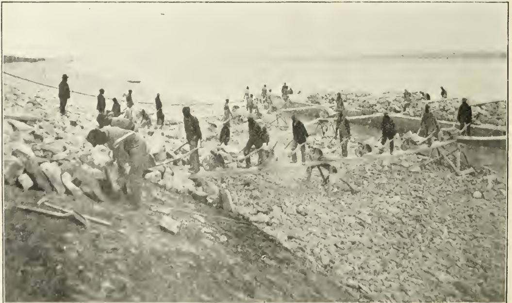
From a] COVERING THE MATS WITH A FACING OF STONES. [Photo.
