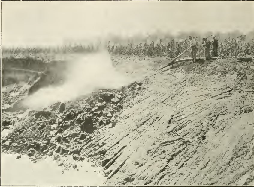
From a] WASHING DOWN EARTH SO AS TO COVER THE MATS AND FORM A "JOINT." [Photo.
