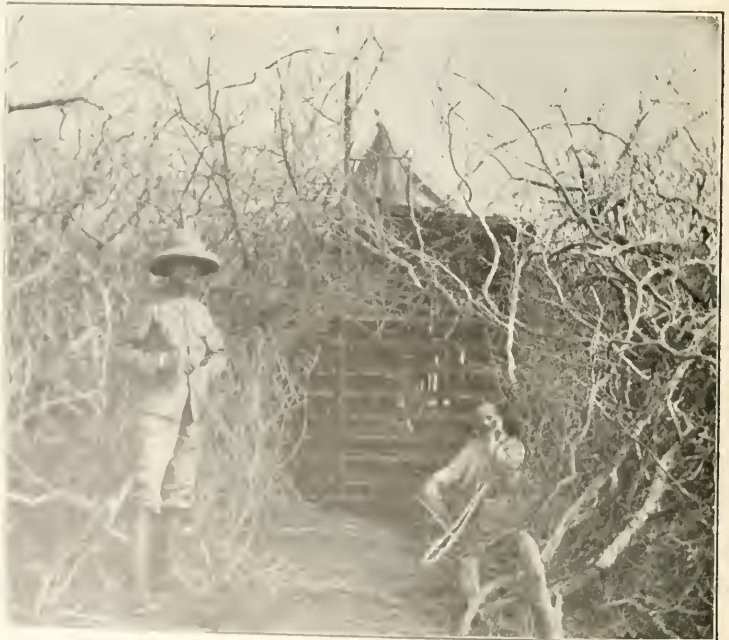
THE TRAM—CONSTRUCTED OF WOODEN SLEEPERS AND TRAM-RAILS. From a Photo.
