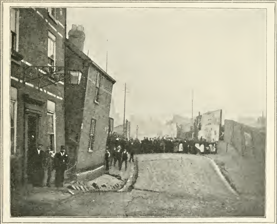
From a THE LONDON ROAD SUBSIDENCE—THE ROAD AS IT APPEARED WITH ITS "BACK BROKEN." [Photo.]
