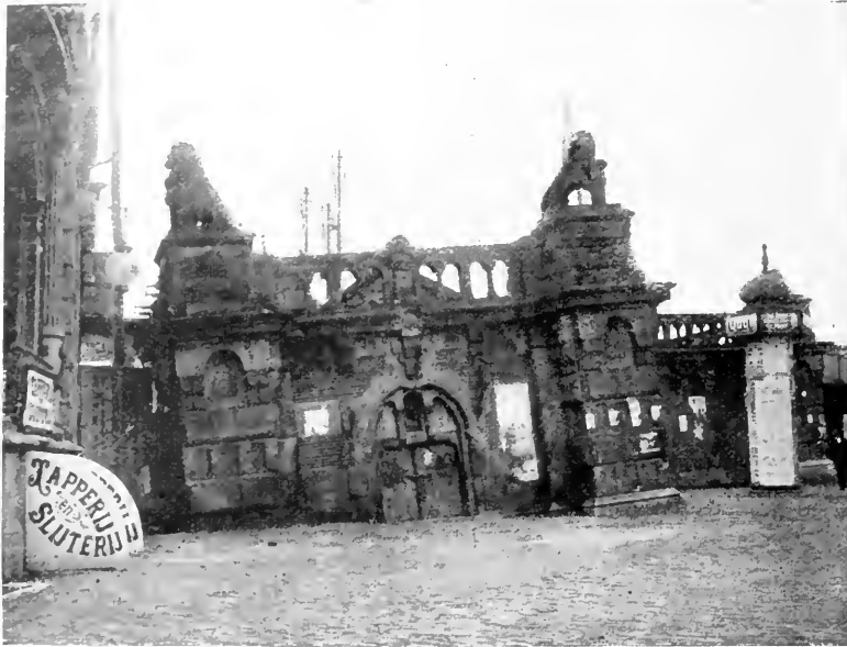
THE RESULT OF A SUBSIDENCE AT THE CENTRAL RAILWAY STATION, AMSTERDAM. [Photo.]
