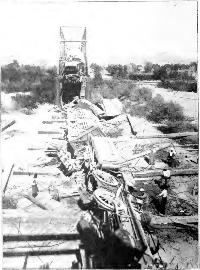
THE BRIDGE, IN ARIZONA, GAVE WAY JUST AS A THE PASSENGER CAR BEING LEFT POISED, HALF ON AND HALF OFF THE BRIDGE. Photo taken by Havstwell and Hamaker, Phoenix.
