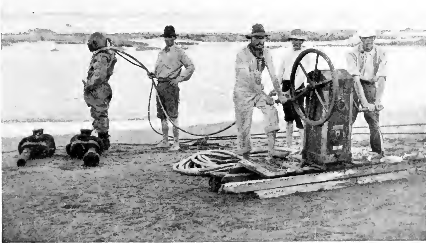
THE DIVER PREPARING TO MAKE A TRIP TO THE WRECK. AT HIS FEET ARE THE VESSEL'S PUMPS, WHICH HE SUCCEEDED IN RECOVERING. [B. W. Camp.]
