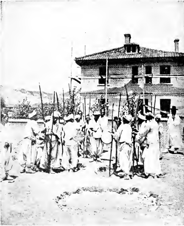
KOREAN LABOURERS AT "WORK"—THEY ARE THUMPING THE GROUND WITH BAMBOO POLES, KEEPING TIME TO THE BEATING OF A DRUM.
