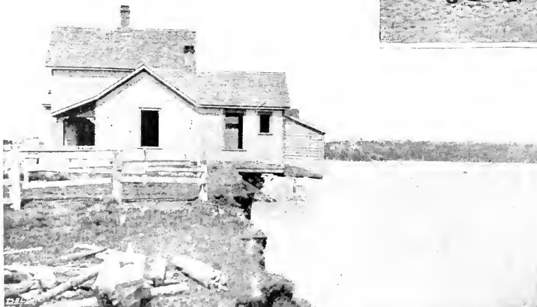
WHAT A FLOODED RIVER CAN DO--THE NIGHT BEFORE THE WATER ROSE THIS HOUSE STOOD FIFTY FEET ABOVE HIGH-WATER-MARK.
