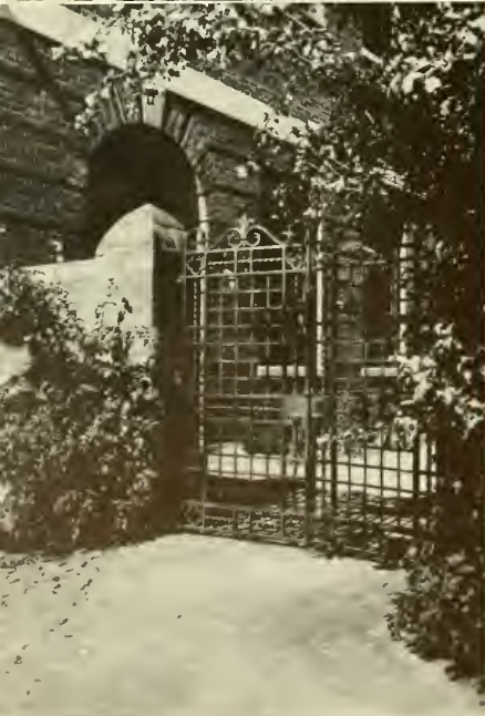
Top: ADMINISTRATION BUILDING
