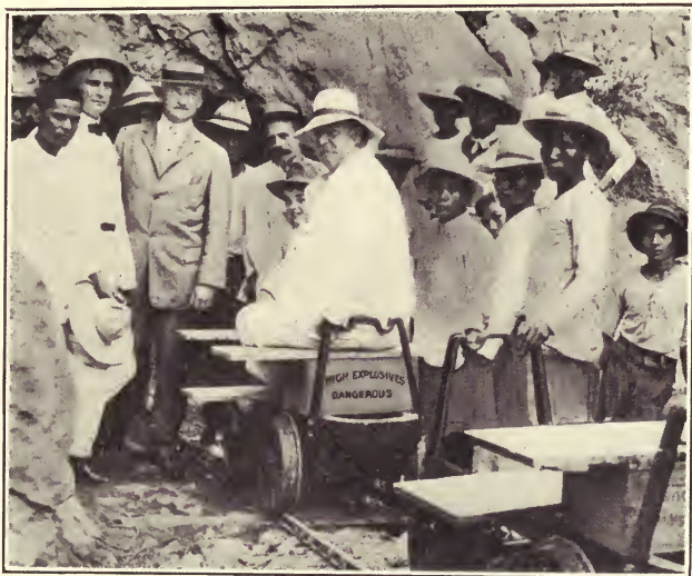
Through the Aqueduct on a Hand Car
