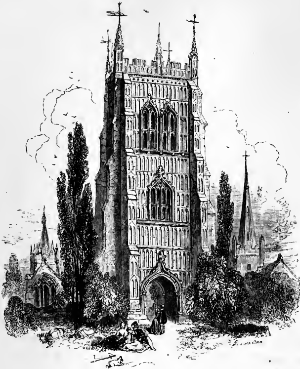
Evesham. The Bell Tower.
