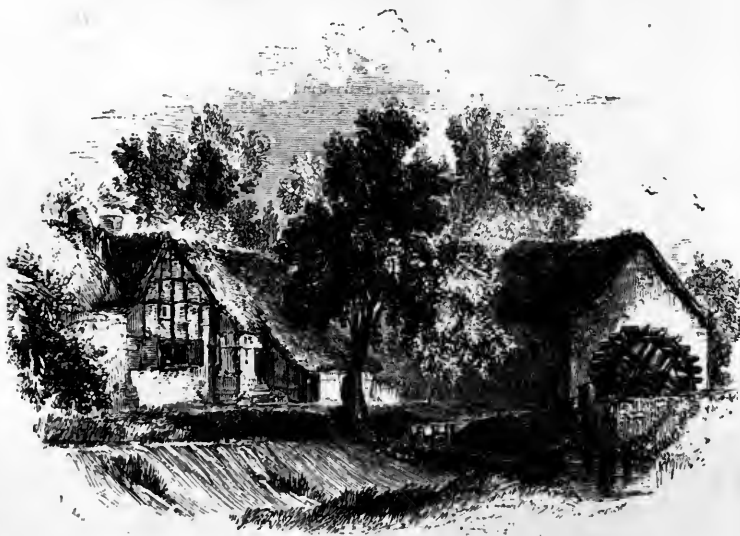
[The Mill; Welford.]
