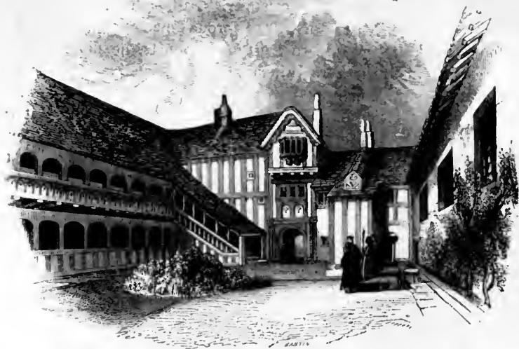
[Leicester's Hospital, Warwick.]
