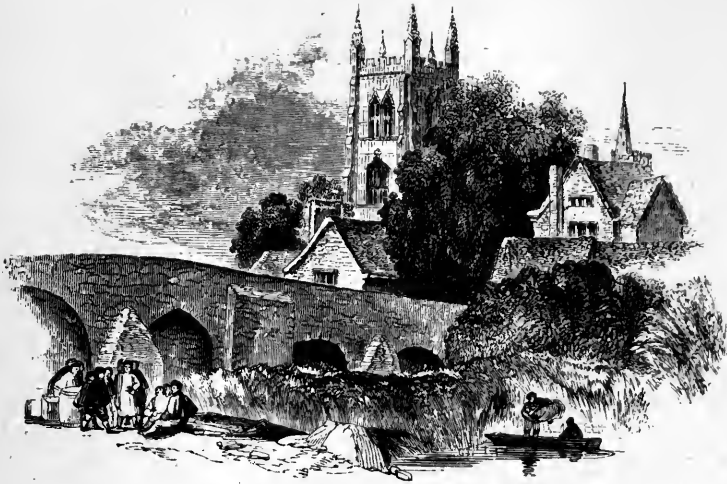
[Bridge at Evesham.]
