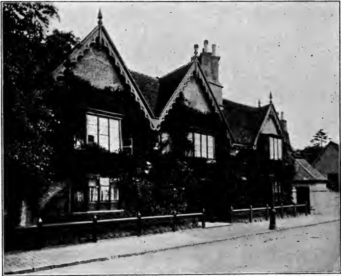
DR. JOHN HALL'S HOUSE AT STRATFORD.
