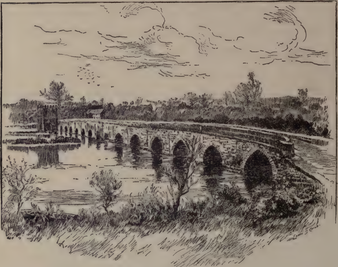
OLD CLOPTON BRIDGE.
