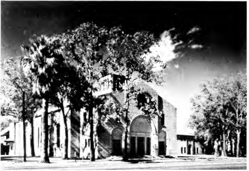
The Central Church of Christ, designed in 1939 and located in the 4100 block of Montrose in Houston, again allowed Watkin to put into practice many of his recommendations from The Church of Tomorrow . Photo by Shoemake-Stiles.
