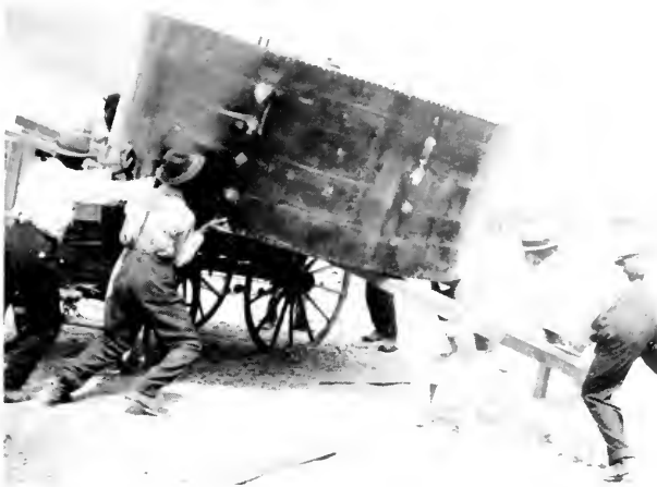
A gasoline tank is put into place for the Power Plant in 1910, using one of the means available at that time—manpower. Courtesy of the Rice University Archives.
