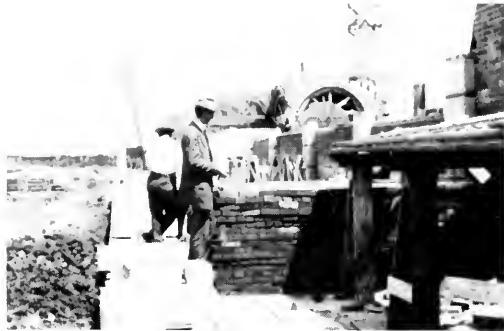
Conducting a test on the cloister slab, south wing of the Administration Building, May 6, 1911. William Ward Watkin is in the coat and hat in the foreground.
