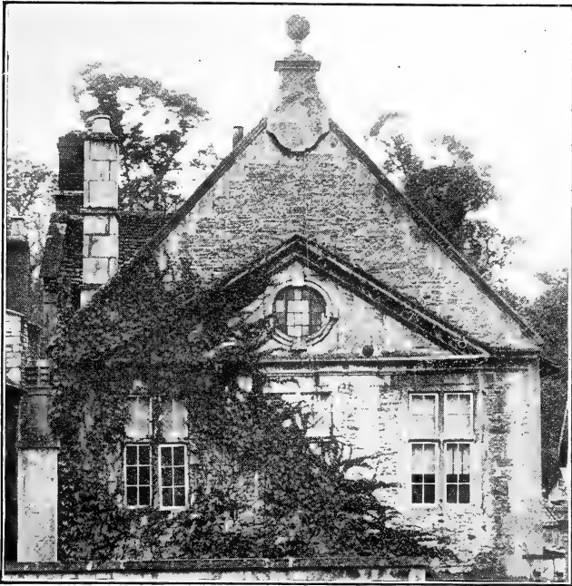
(1).—Corsham. The W. Gable of the old Poor House.
