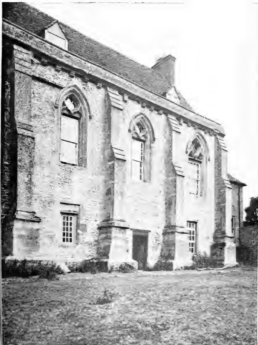
Fig. 4.—Bradenstoke Priory, south end of western range.
