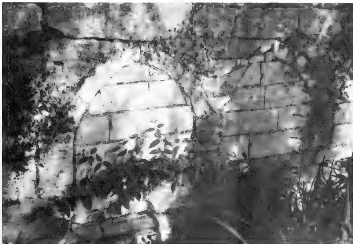
Figure 7. 5 St Margaret's Place, Bradford-on-Avon. A set of now blocked-in bee boles, with stone arches in a coursed stone wall. The only arched example found in stone.
