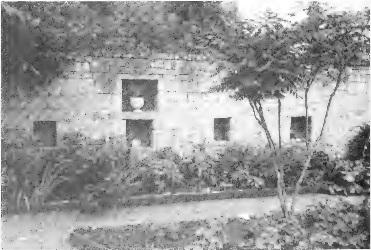
Figure 4. The Wilderness, Box. Rectangular boles with stone lintels in ashlar stone wall. This is the simplest type of stone bee bole seen, with variations, at 6 of the 13 Wiltshire sites.
