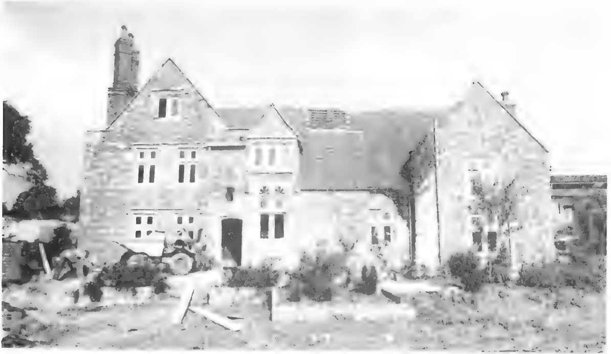
Figure 1. Manor House, Upton Scudamore, from the S during renovation in 1985.
