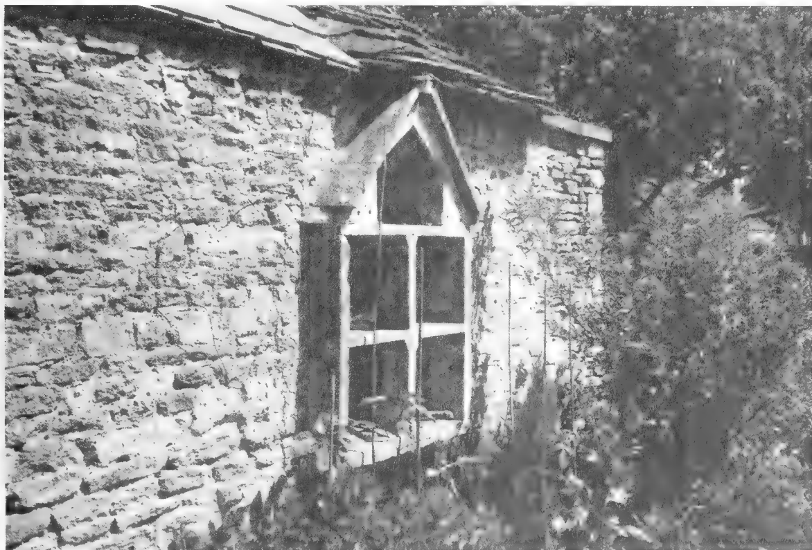
Figure 5. Little House, Biddestone. An elaborate gabled set in stone. The example from neighbouring Honeybrook Farm is almost identical. Note the boles in the projecting side walls, perhaps to hold a bar to secure the skeps.
