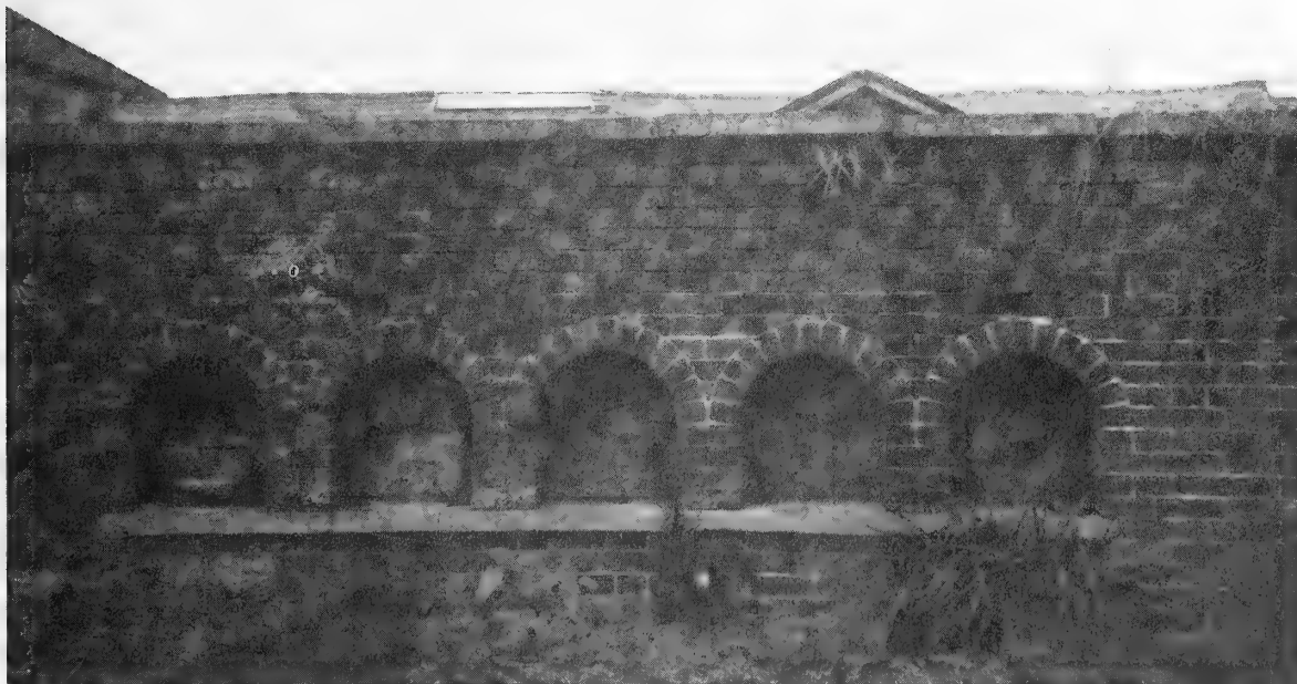
Figure 3. Widbrook Farm, Bradford-on-Avon. Set of 5 brick bee boles in a wall flanking the house. The two other sets in brick (Littleton House and St Denys Convent) are similar but larger, perhaps to hold more than one skep/bole.
