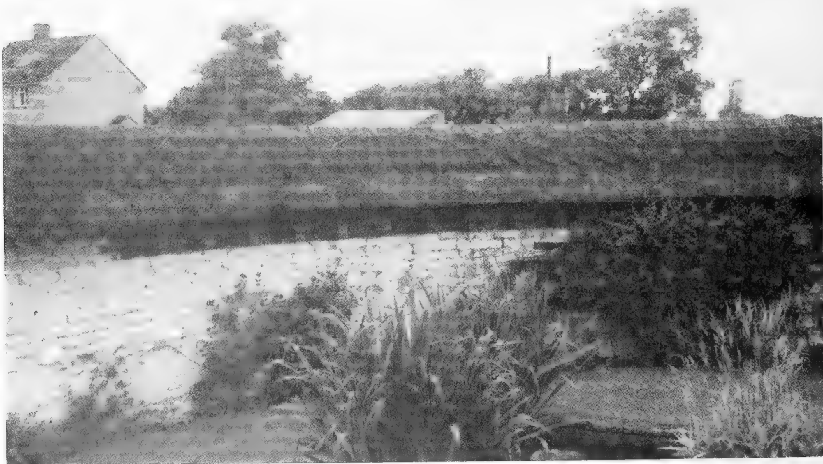
Figure 6. Uffcott Farm, Broad Hinton. A unique set of 20 bee boles in a wall of chalk blocks. The boles are defined by brick piers.
