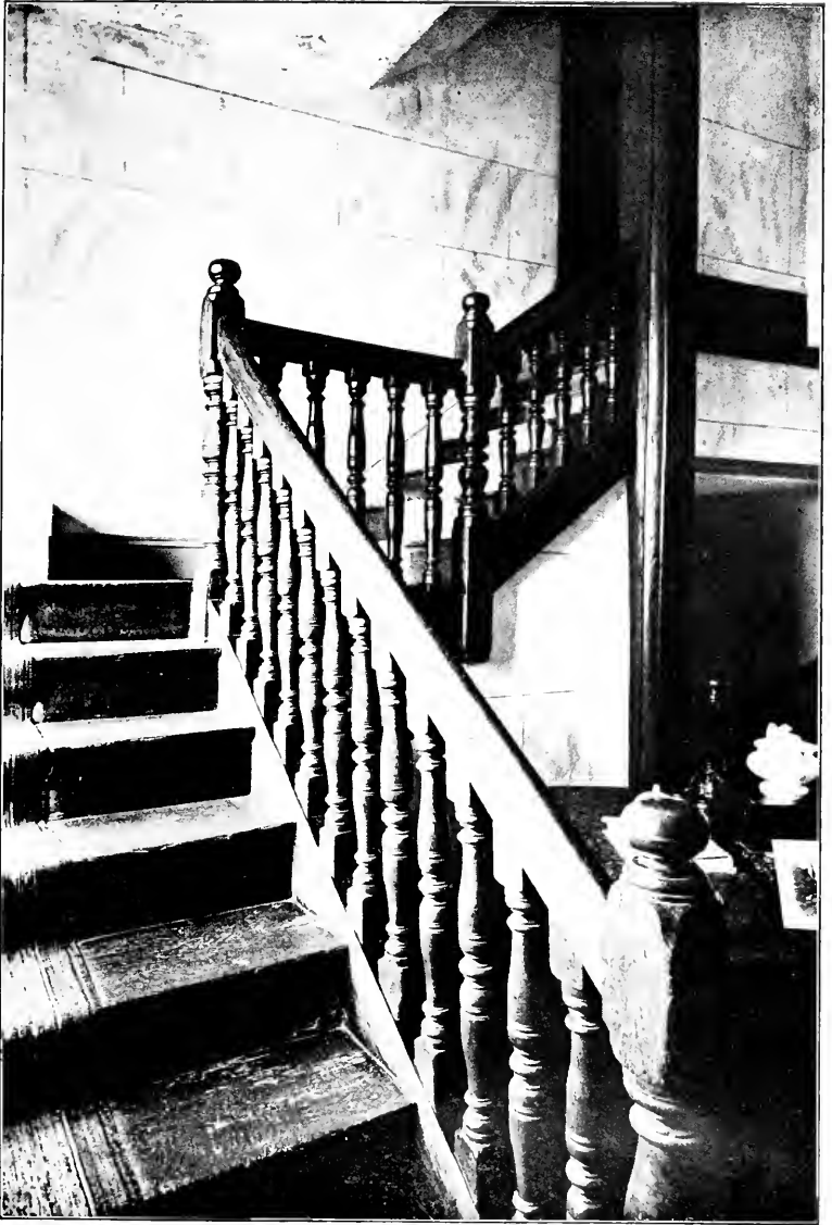
STAIRCASE AT GARSDON MANOR HOUSE. (Lower Portion.)
