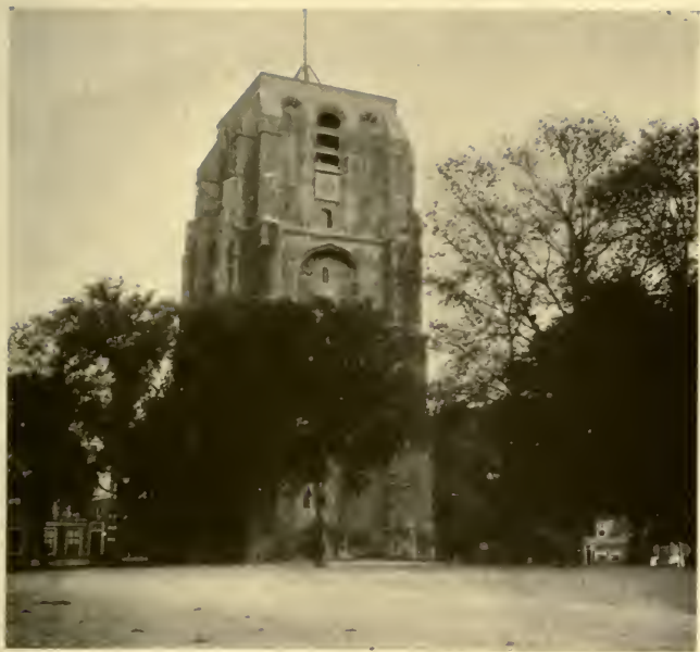
Leeuwarden's structural curiosity is the Olde-Hove, an unfinished church tower of brick, leaning with all the abandon of Pisa's Tower
