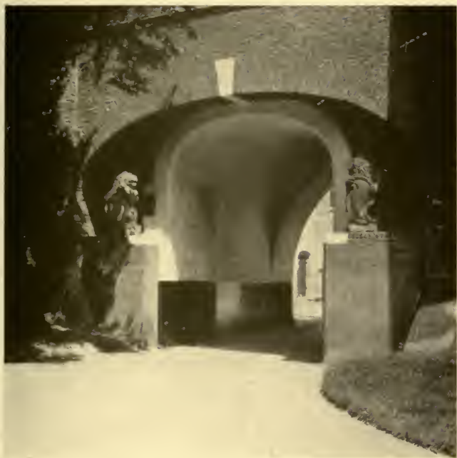
The best of Kampen's gateways, of which architectural features the town originally possessed seven
