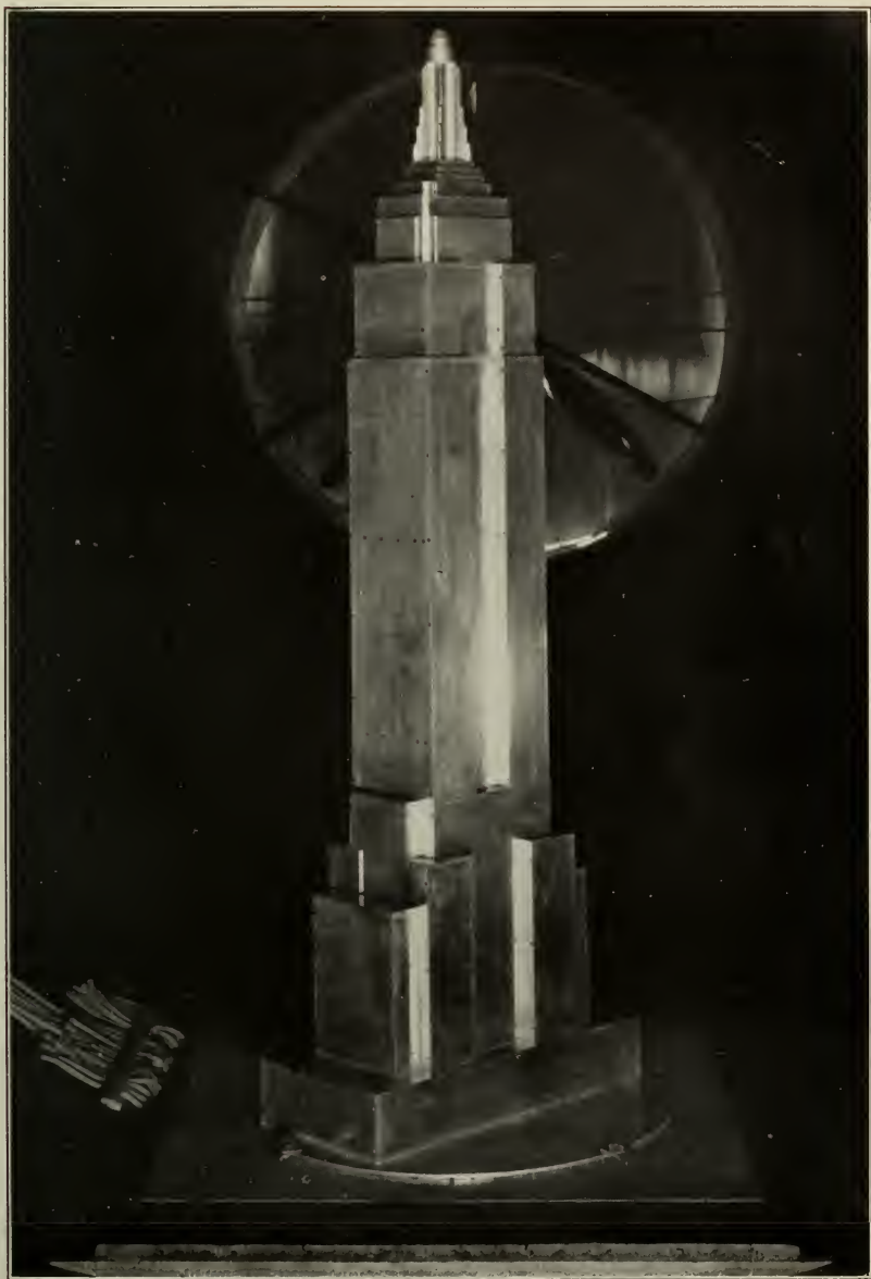
FIGURE 1.— Model of the Empire State Building in the wind tunnel, looking downstream
