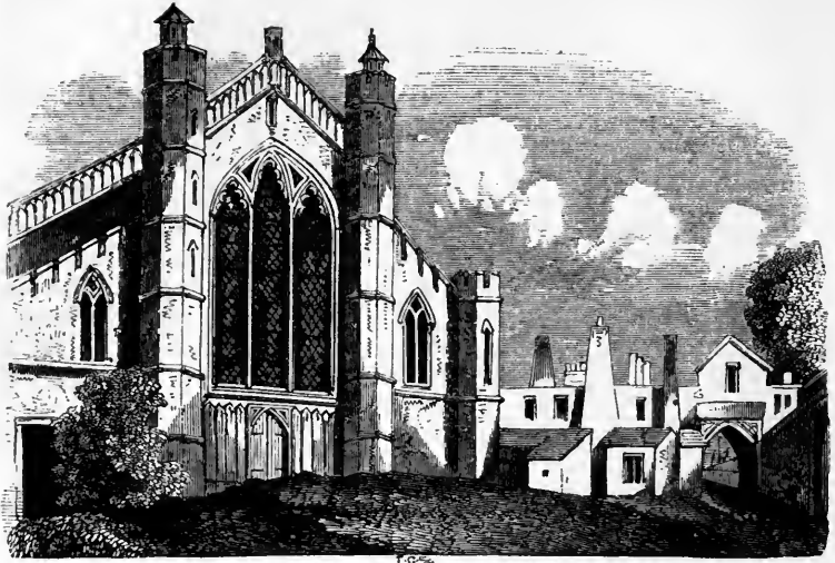
WEST END OF SAINT GEORGE'S CHAPEL
