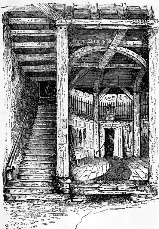
INTERIOR OF THE CURFEW TOWER.
