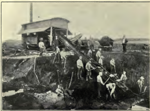
FIG. 1.—ANREP-SVEDALA. ELEVATOR AND MACERATING MACHINE.
