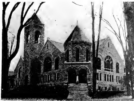
Methodist Episcopal Church nearing completion—Photo by K. T. Sheldon
