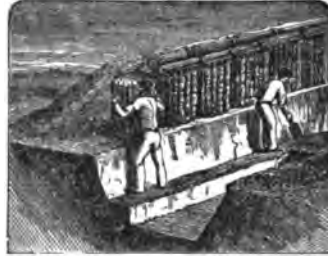
Part of Trench with Gabions and Fascines.
