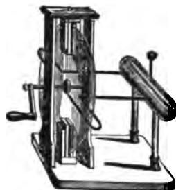
Fig. 2.—Plate Electric Machine.
