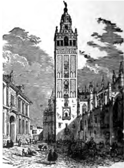
Seville.— La Giralda and part of the Cathedral.
