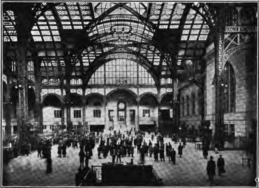
THE CONCOURSE PENNSYLVANIA RAILROAD STATION
