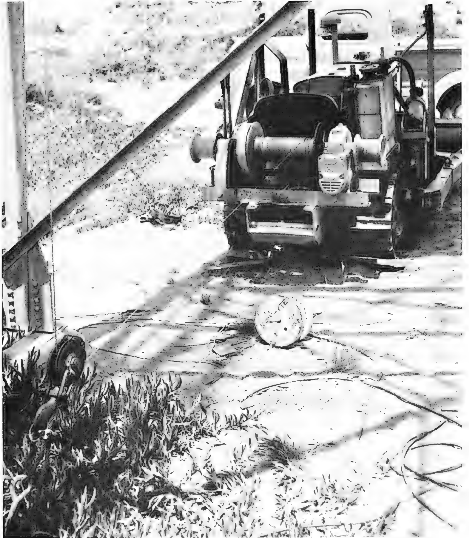
Figure 2. Tractor and winch used for raising and lowering test cable.
