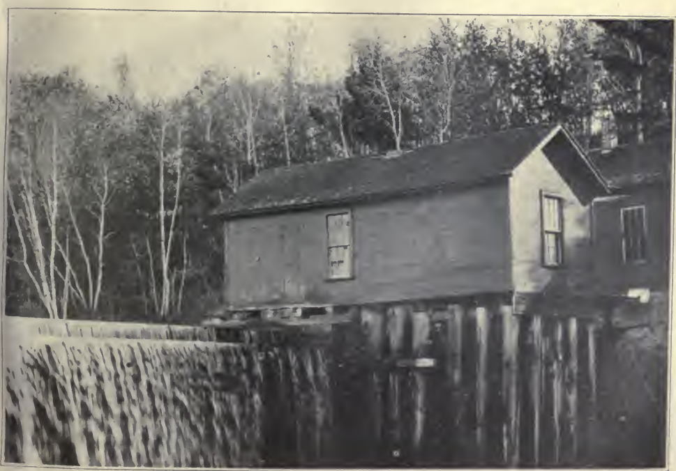
THE BURKHARDT MILLING AND ELECTRIC POWER PLANT
