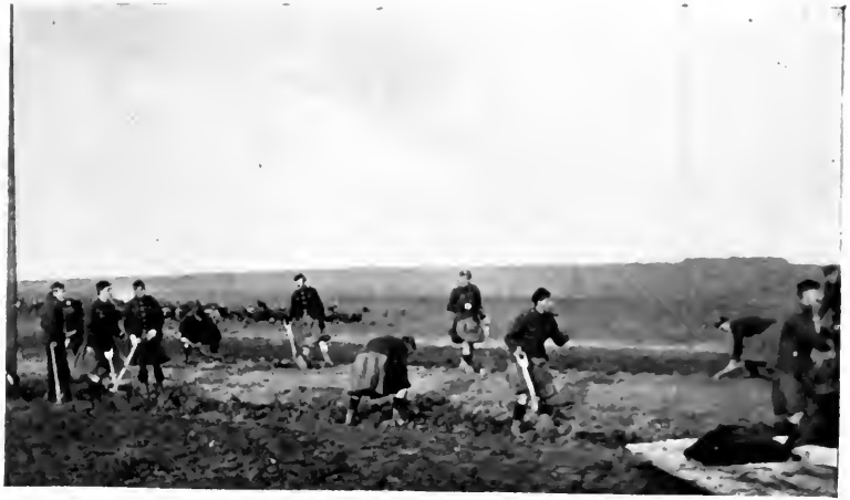
DIGGING TRENCHES—SALISBURY PLAIN.
