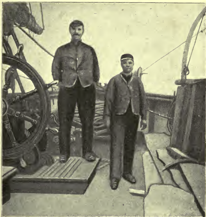
JOHANSEN AND PETTERSON AFTER CLEANING THE BOILERS.
