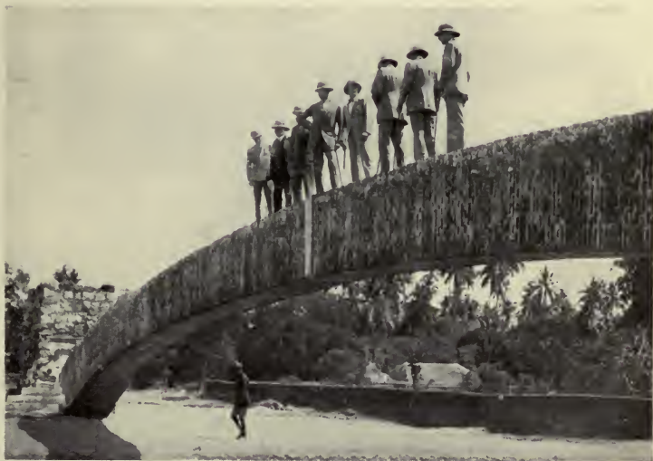
THE PRINCE AND HIS STAFF AT SERINGAPATAM TESTING A BRICK SPAN INVENTED BY COL. HAVILAND TO ENABLE TROOPS TO CROSS THE NUMEROUS WATERCOURSES
