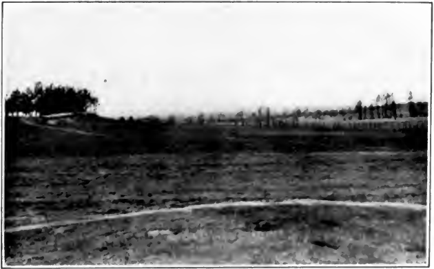
PREPARED RESERVE TRENCH
