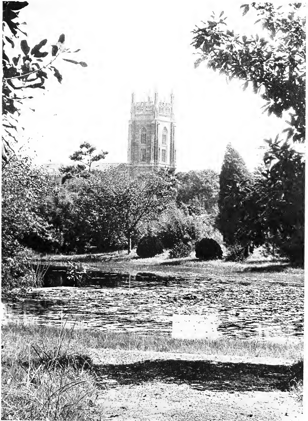
Chapel Tower From Park
