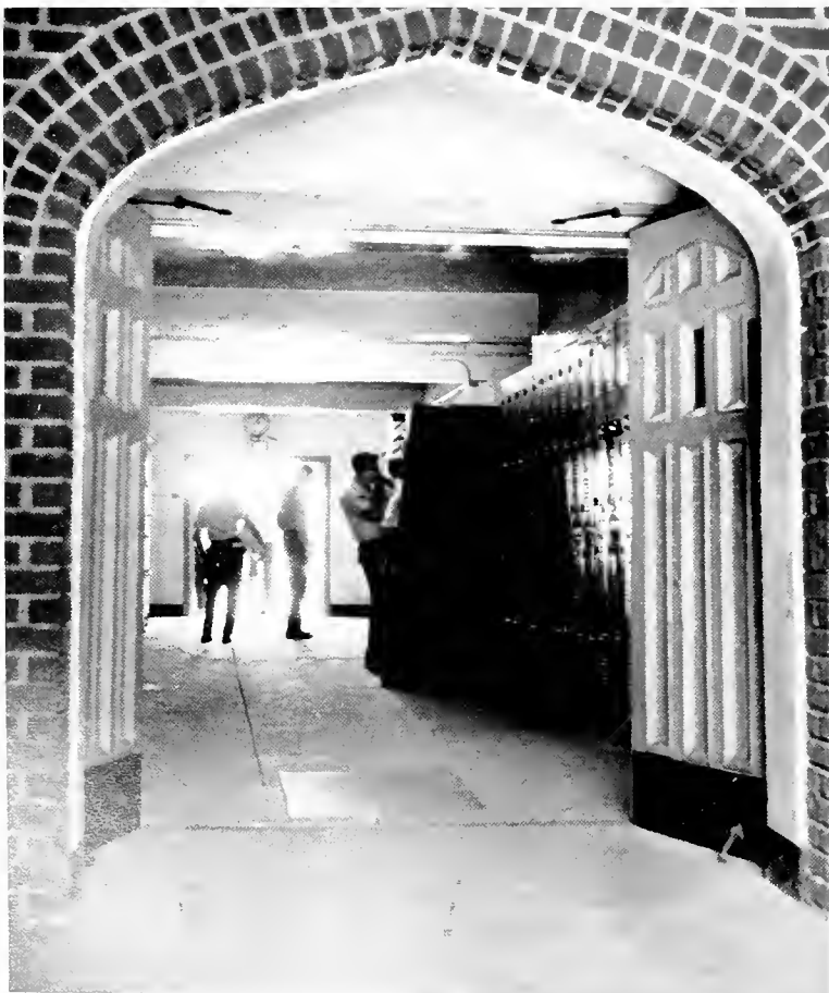
Workman's eye view of Marquette hall as seen from the air conditioning plant's construction site.
