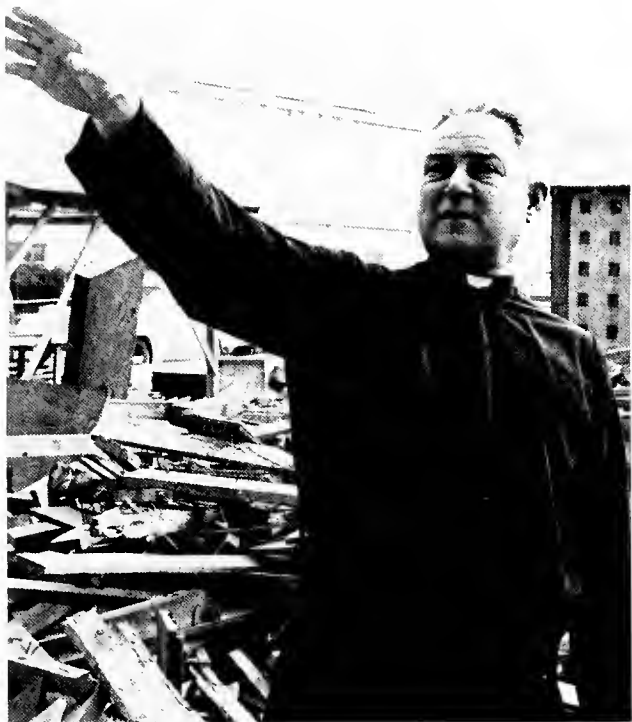
After an inspection tour of worker progress on the new student center Father Doyle talks over the future plans for the buildings with Father Smith.
