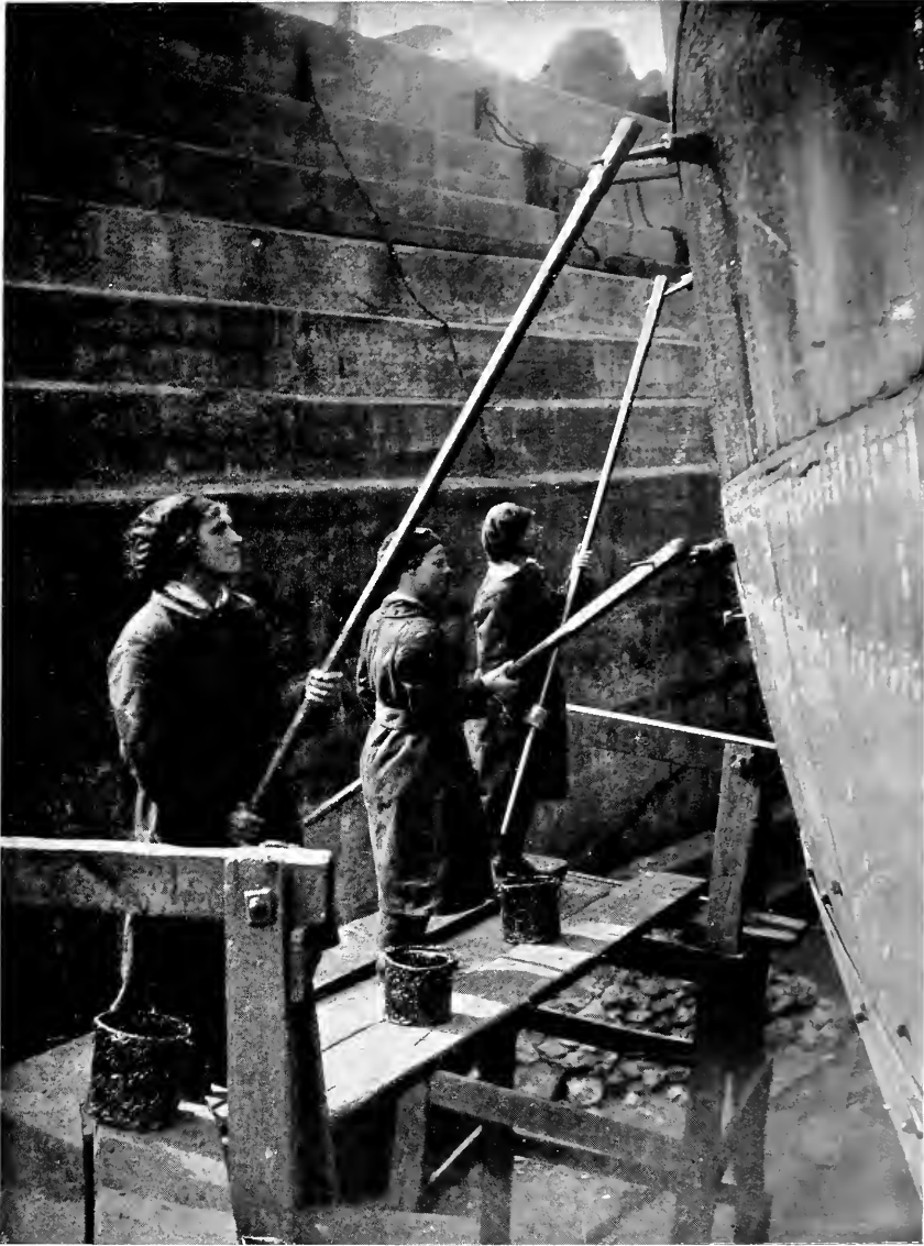
PAINING A SHIP'S SIDE IN DRY DOCK
