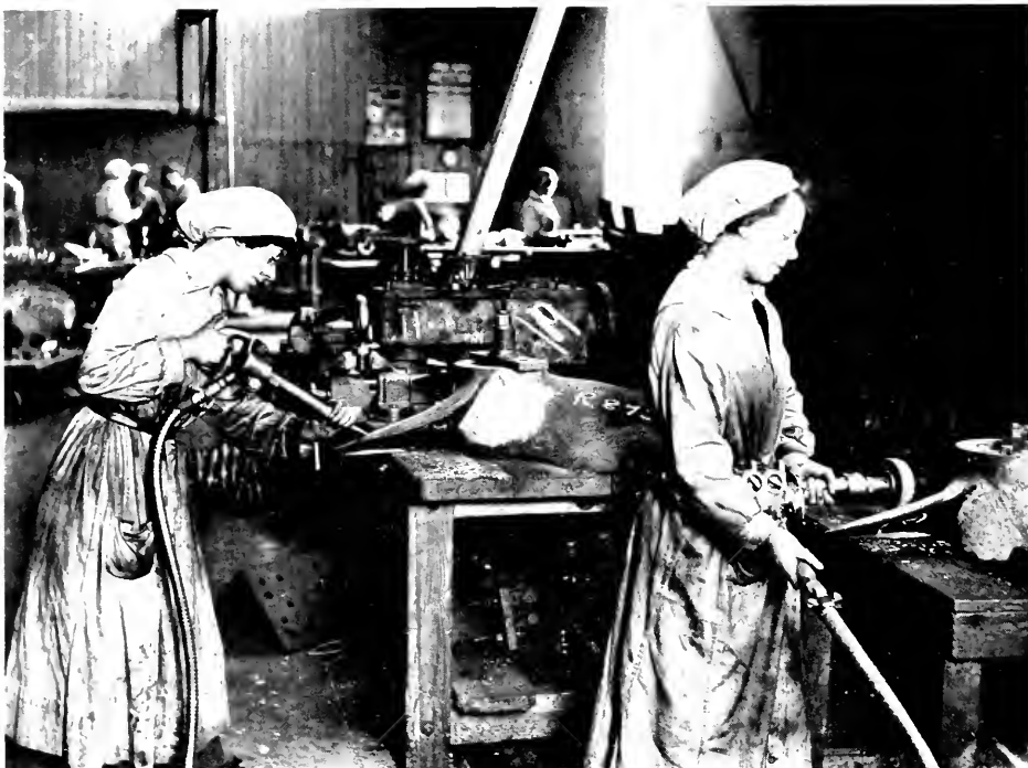
CHIPPING AND GRINDING BLADES OF CAST IRON PROPELLER WITH PORTABLE TOOLS
