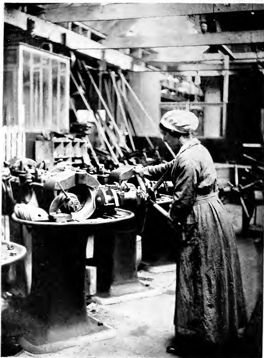
OPERATING A LUMSDEN PLAIN GRINDER: RE-FORMING 8-INCH HIGH-EXP LOSIVE CUTTERS
