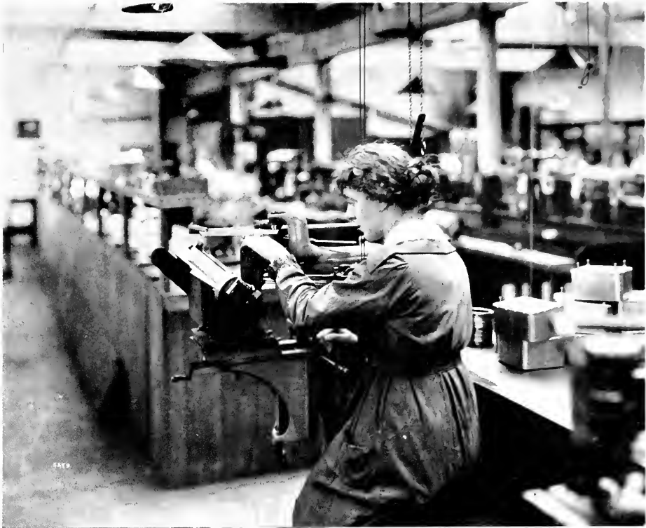
ENGRAVING METAL PARTS FOR COMPASSES
