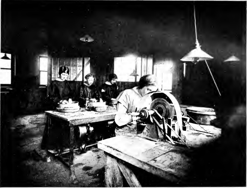
SLITTING AND ROUGHING OPTICAL GLASS
