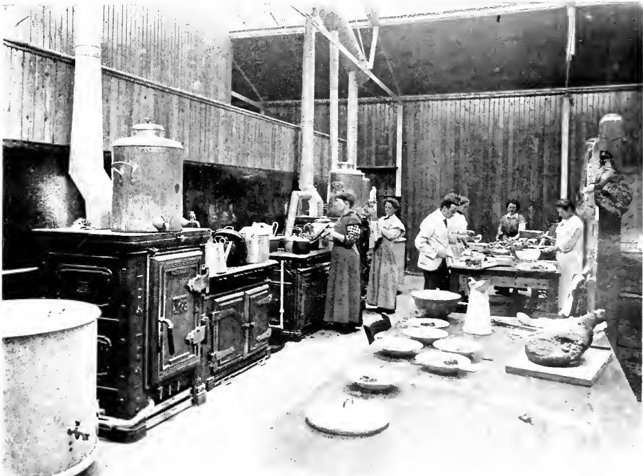
VIEW OF CANTEEN KITCHEN
