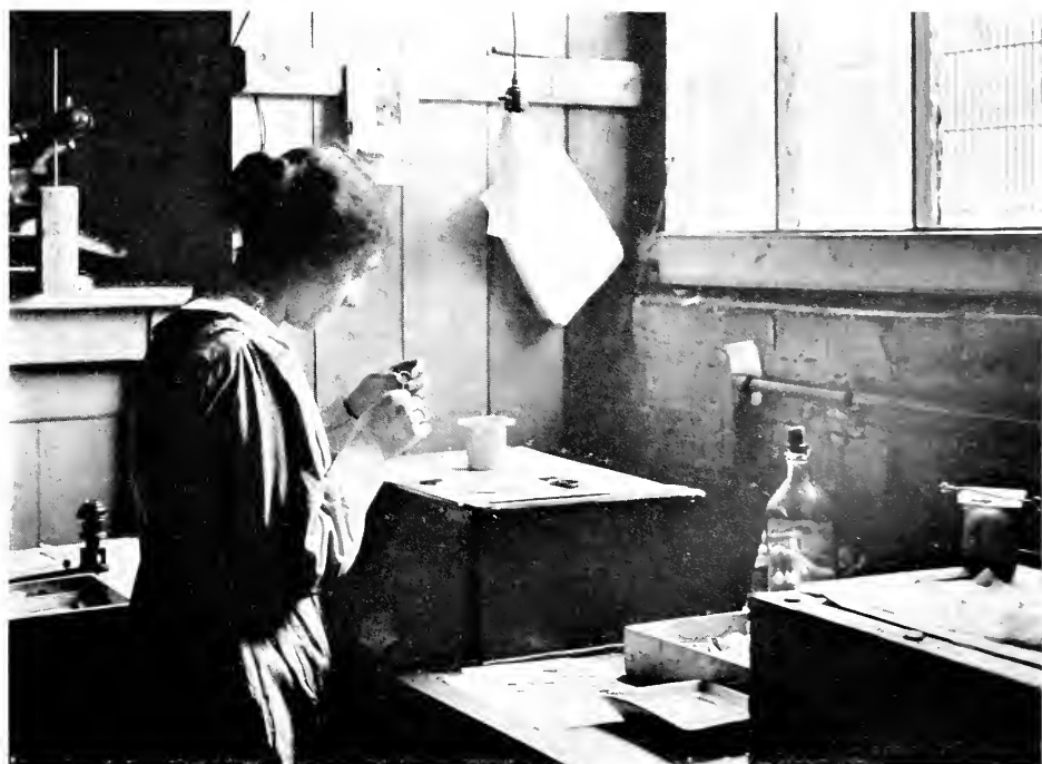
BRAZING TURBINE ROTOR SEGMENT
