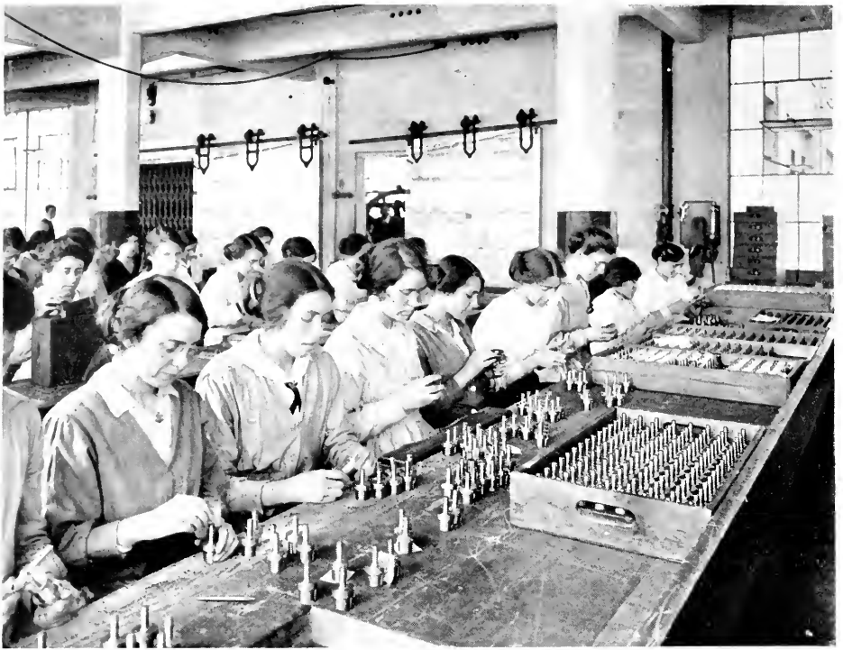
INSPECTING AND GAUGING FUSES
