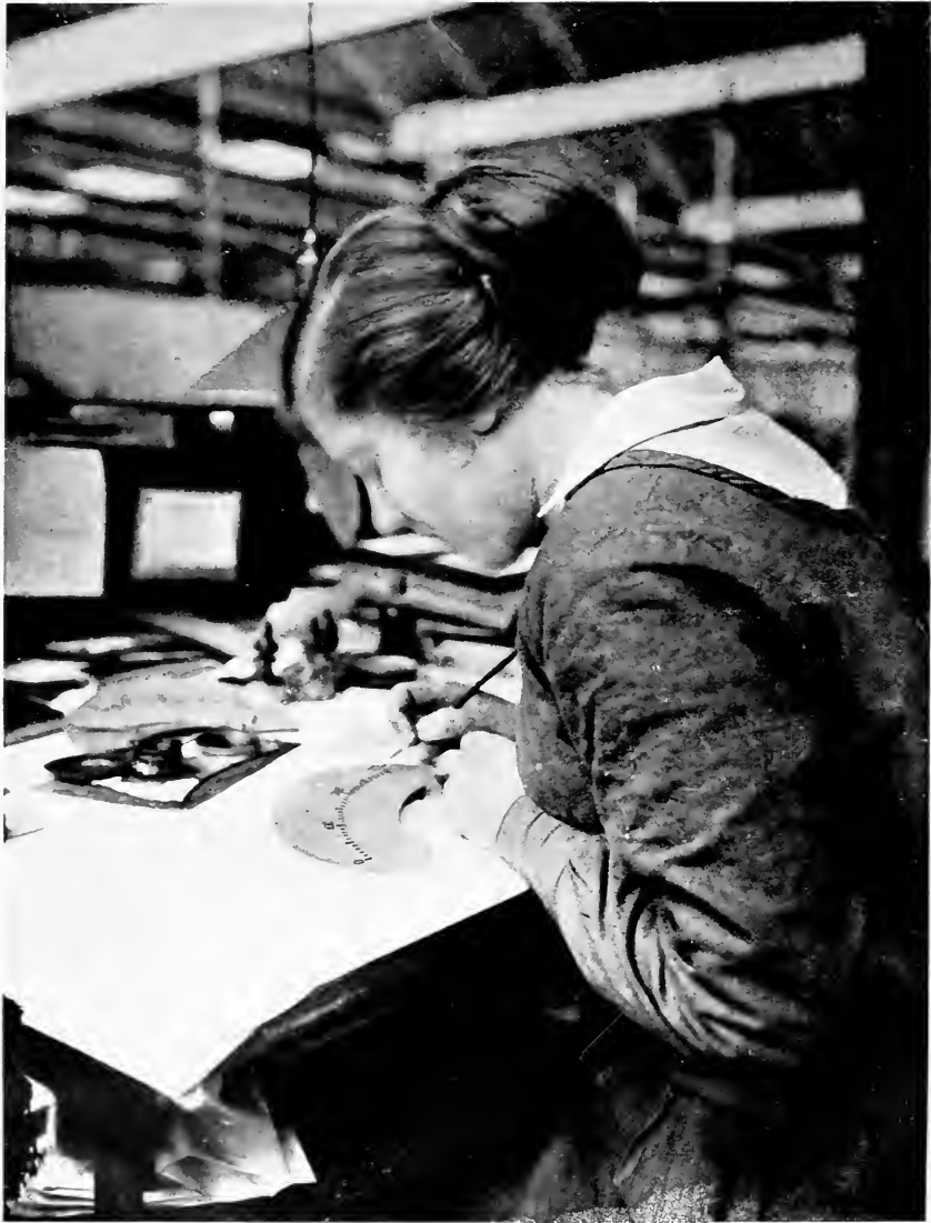
MAKING INSTRUMENT SCALES
