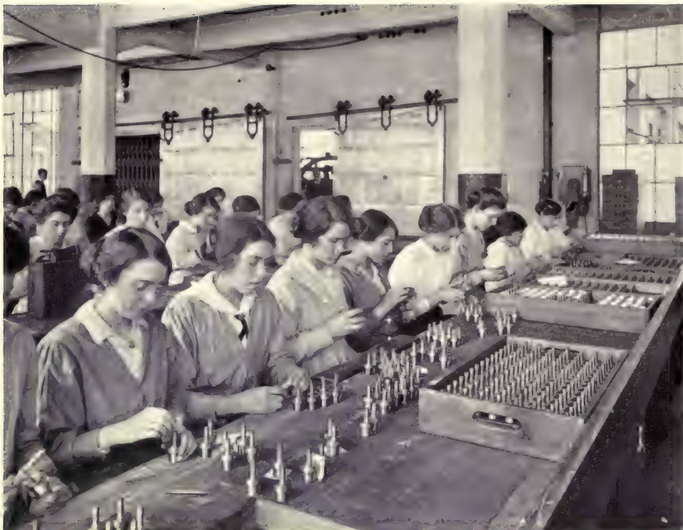
INSPECTING AND GAUGING FUSES
