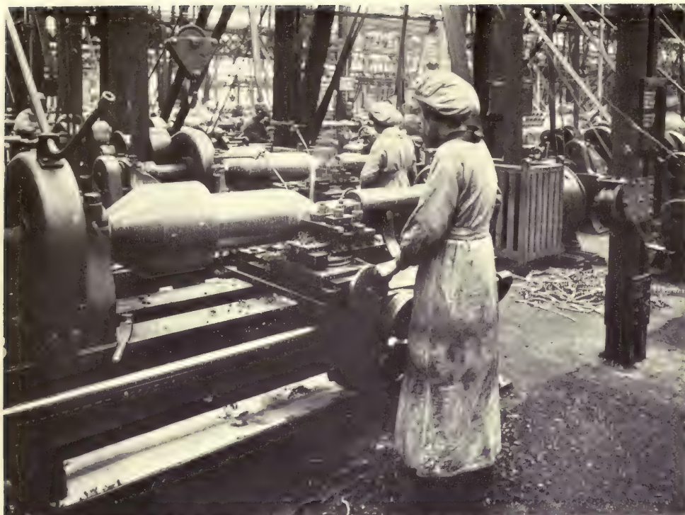
TURNING THE COPPER BAND OF A 9.2-INCH HIGH-EXPLOSIVE SHELL
