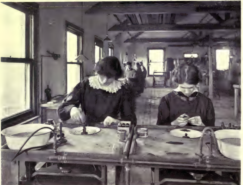
TREADLE POLISHING-MACHINES, FOR SMOOTHING LENSES
