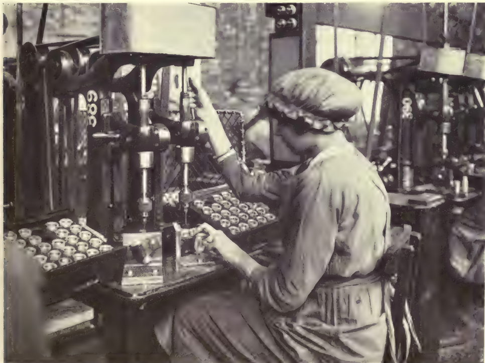
DRILLING SAFETY-PIN HOLE IN FUSE
