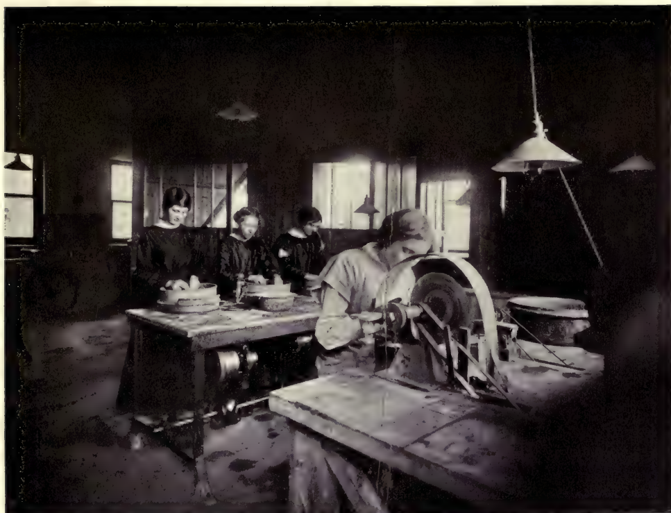
SLITTING AND ROUGHING OPTICAL GLASS
