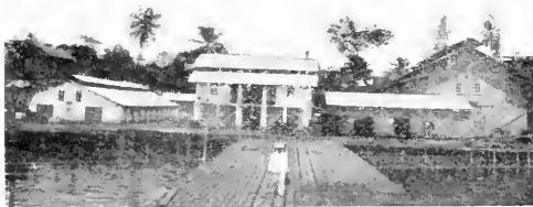
LANDING PIER, DUALA.
