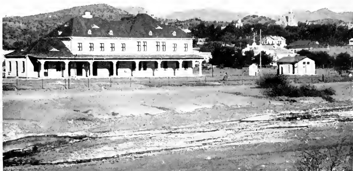
RAILWAY STATION, WINDHUK.
