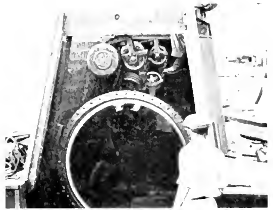
THE OPERATING CHAMBER BEING LOWERED INTO THE WATER.
