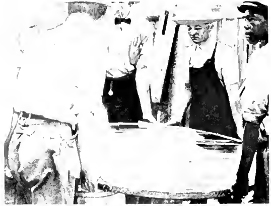
PLACING IN POSITION THE HUGE CIRCULAR GLASS PLATE WHICH FORMED THE WINDOW OF THE OPERATING CHAMBER.
