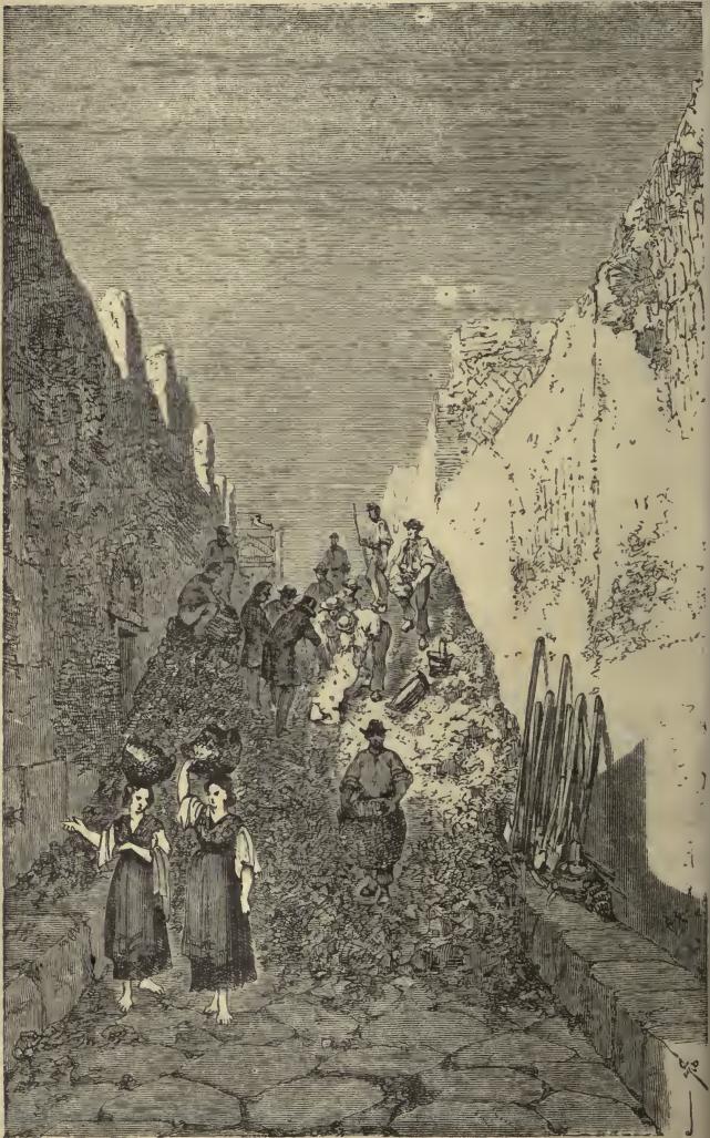
Clearing out a Narrow Street in Pompeii.
