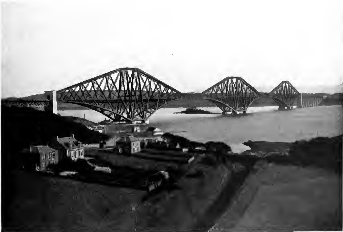
THE FORTH BRIDGE, SCOTLAND.
