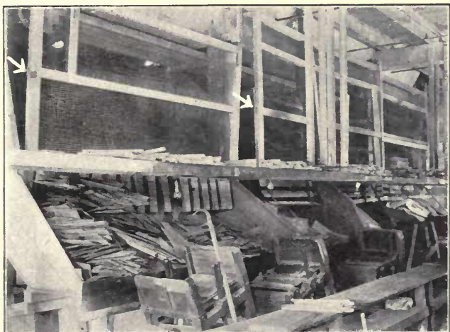
Fig. 72. Screen and Guards for Shingle Packers.
