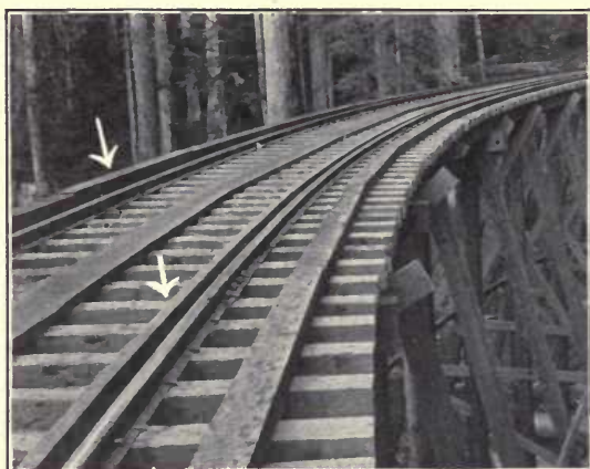
Fig. 2. Trestle with Guard Rails and Walks.
