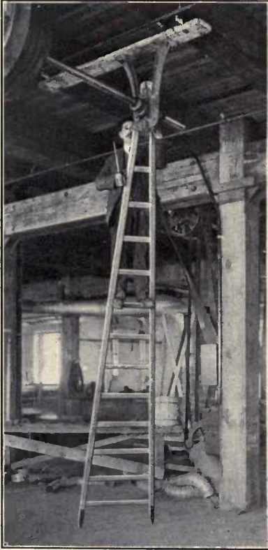
Fig. 306. Triangular Ladder with Steel Points at Bottom.
