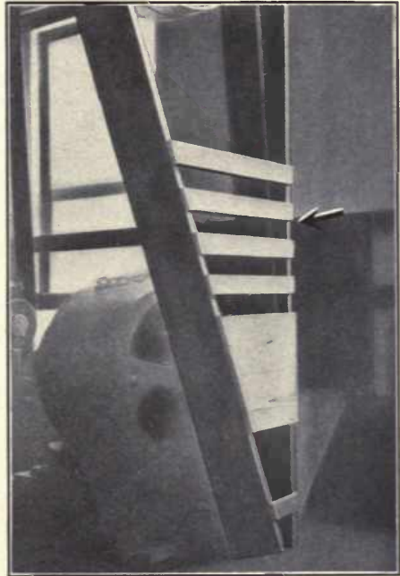
Fig. 297. Guard for Motor Belt near Passageway.
