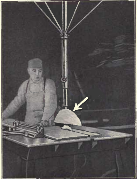
Fig. 95. Adjustable Hood Guard.
