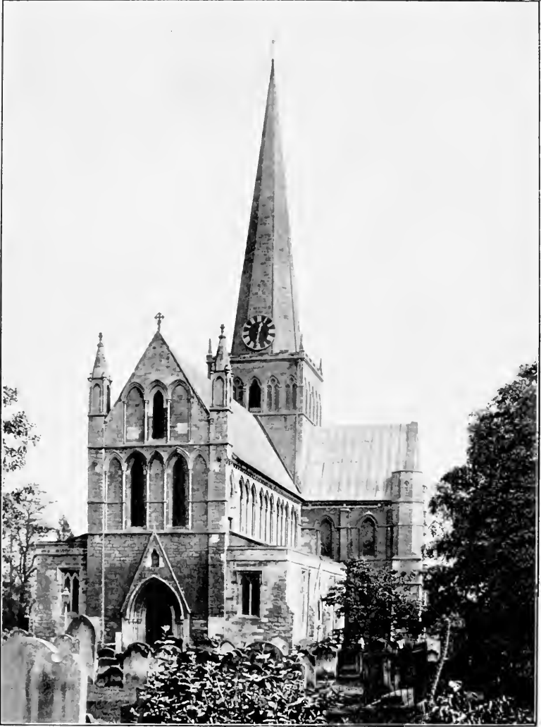
ST. CUTHBERT'S CHURCH FROM SOUTH-WEST.
