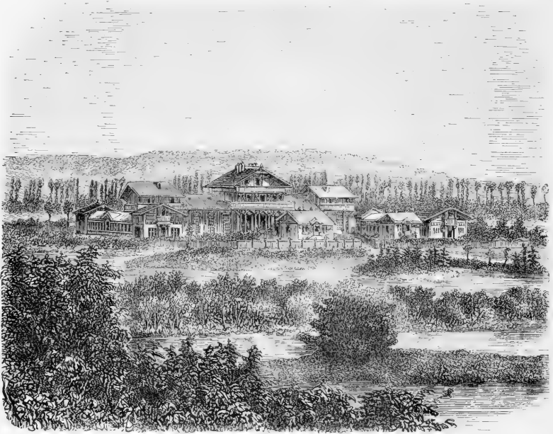
GENERAL VIEW OF THE PISCICULTURE ESTABLISHMENT AT HUNINGUE.
