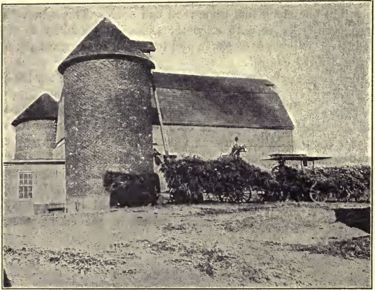
FIG. 45.—Barn with masonry silos. The chopped corn goes up the pipe by air pressure. (U. S. Dept. Agr.)
