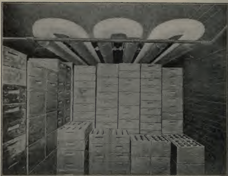
FIG. 85.—Ammonia pipes cooling a car for the shipment of milk to market. (U. S. Dept. Agr.)
