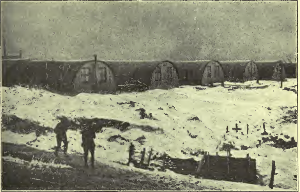
PORTABLE HOUSES, ON THE FRONT, CALLED NISSEN HUTS
