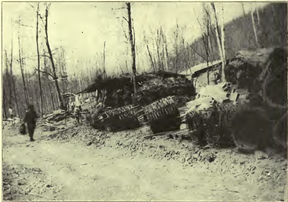
A FIELD FORTIFICATION SUPPLY POST
