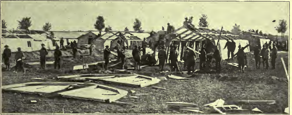
ENGINEERS ERECTING A CANTONMENT IN FRANCE
