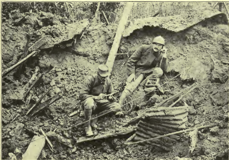
A COMPLICATED SYSTEM OF WIRE AND CABLE
