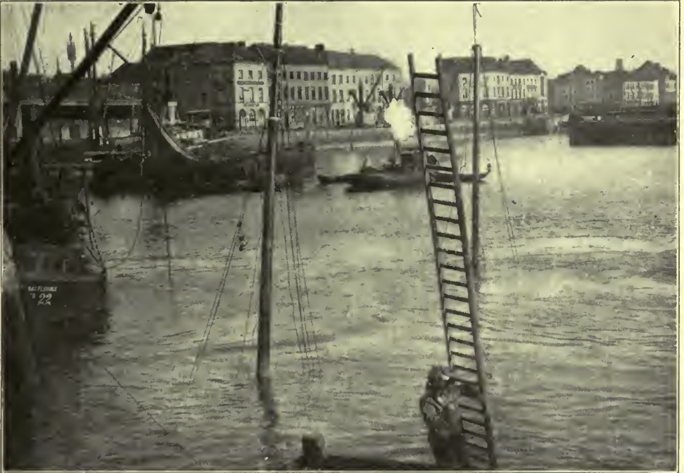
SALVAGING AND CLEARING IN THE HARBOR
