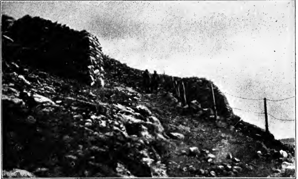
SAND-BAG TRENCHES ON THE CARSO TABLELAND
