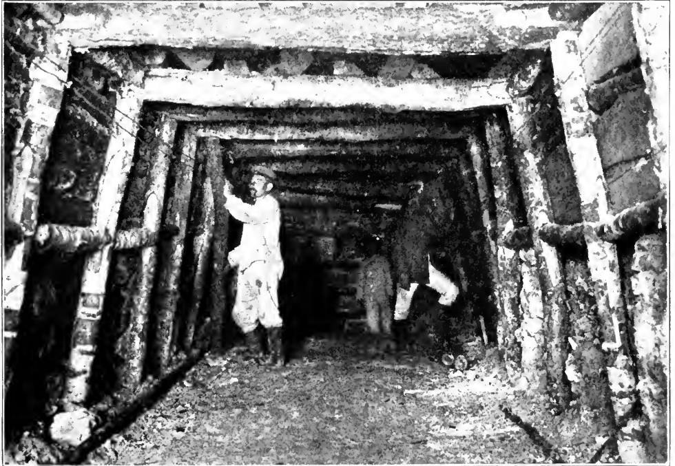
GERMANS AT WORK ON AN UNDERGROUND GALLERY
