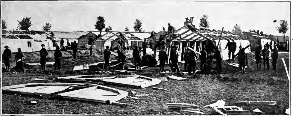
ENGINEERS ERECTING A CANTONMENT IN FRANCE
