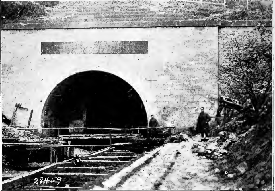
THE SOUTH PORTAL OF THE ST. QUENTIN CANAL
