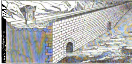
Construction of a Portion of the Appian Way.
