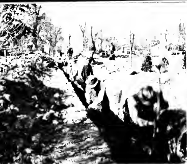
DIGGING UP THE WALKS
