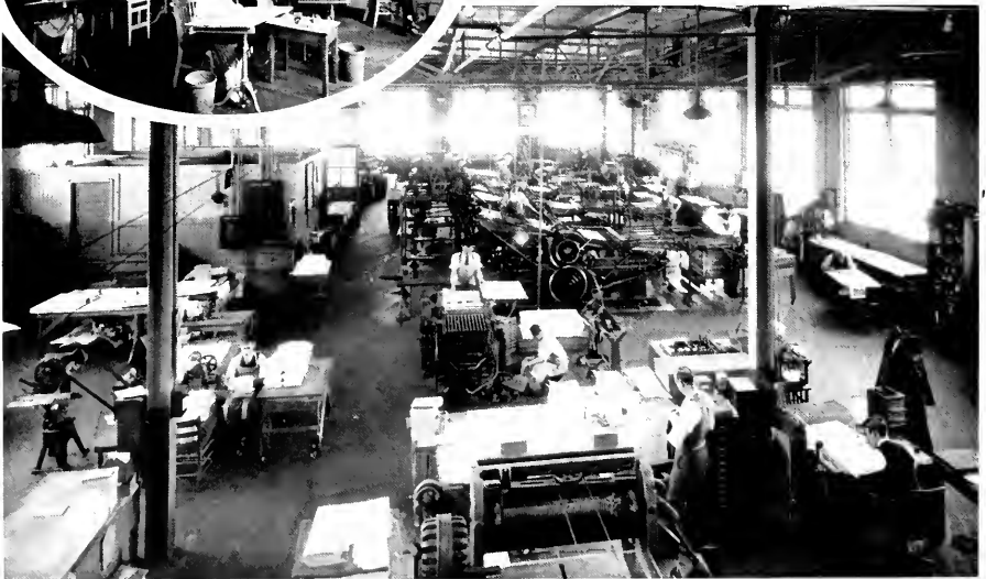
Several Interior Views of Our Modern Plant
