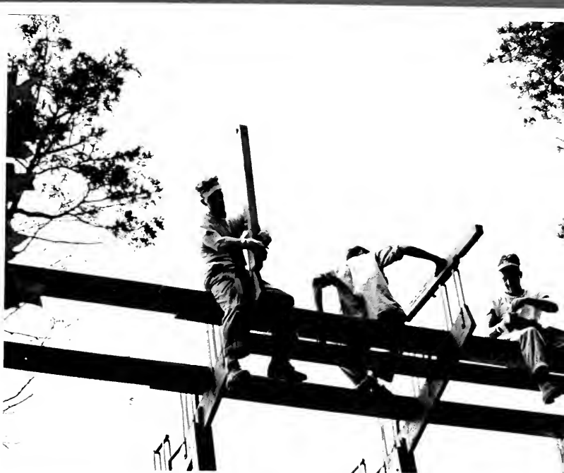
Football players erect stands in Kenan Stadium in preparation for the fall season of sports.
