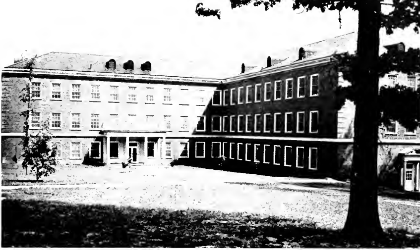
Housing the undergraduate and graduate programs in Dentistry as well as the training facilities for Dental Hygiene, the new building of the School of Dentistry, completed in 1952, is an integral part of the total physical and educational structure of the Division of Health Affairs.
