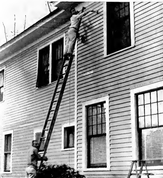
"That's a nice pose . . . now you can come down!"
